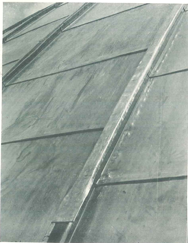
Above: Construction detail of the lead-covered dome of the New Jersey State Reformatory at Rahway, N. J. All seams shown, including those where the sheets join the batten caps, are loose-locked to provide for expansion and contraction.
