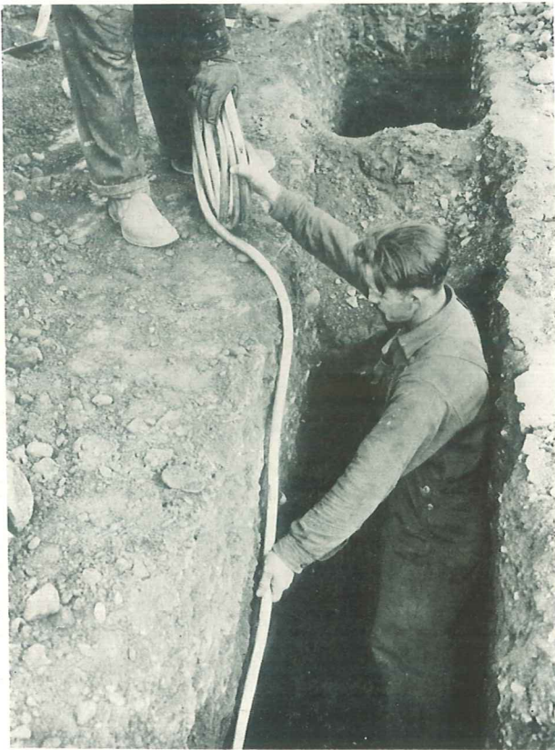
Above: Uncoiling lead pipe in a trench before attaching to water main. Below: Bending lead pipe. Note the bending spring inserted in the pipe. Right: A graphic illustration of lead's flexibility and the advantage taken of it by a skilled plumber.
