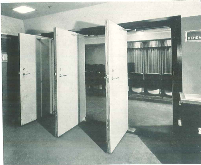
Left: These doors to an N. B. C. broadcasting studio, made from layers of wood and sheet lead, are said to reduce noise by an average of 39.56 decibels.
