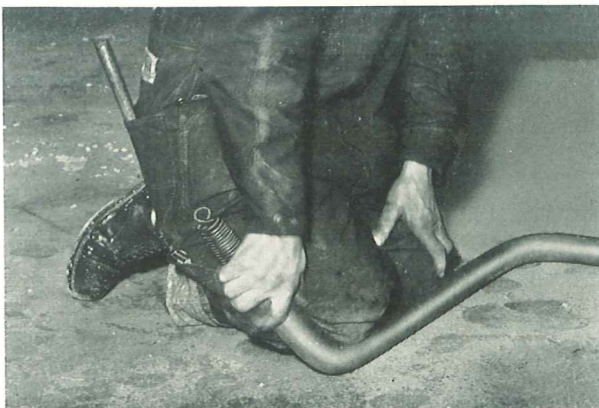
Above: Uncoiling lead pipe in a trench before attaching to water main. Below: Bending lead pipe. Note the bending spring inserted in the pipe. Right: A graphic illustration of lead's flexibility and the advantage taken of it by a skilled plumber.
